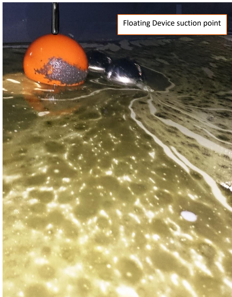
Floating device located inside Coolant Tank.
